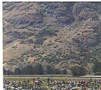
embankment - queenstown cricket ground
